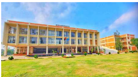
Present view of Academic & Admin Building
