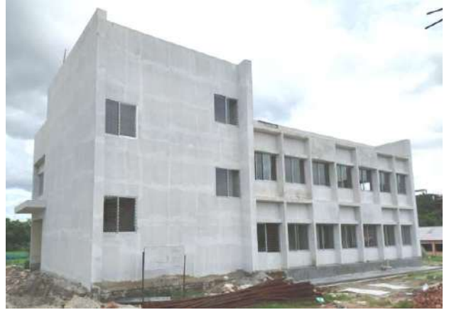
International Hostel Cum Dining Bldg
