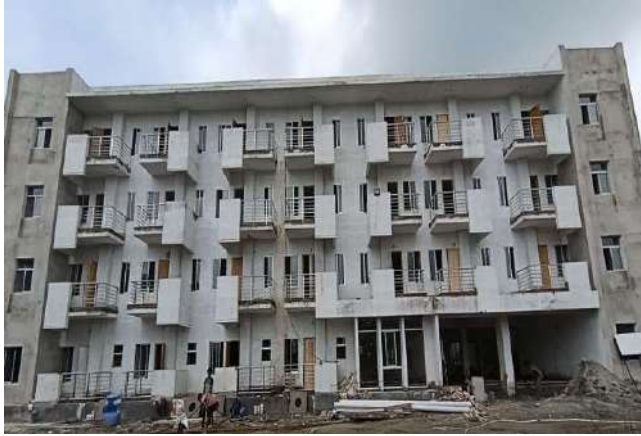
Male Dormitory Bldg
